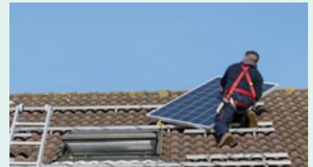
Rooftop solar installation
