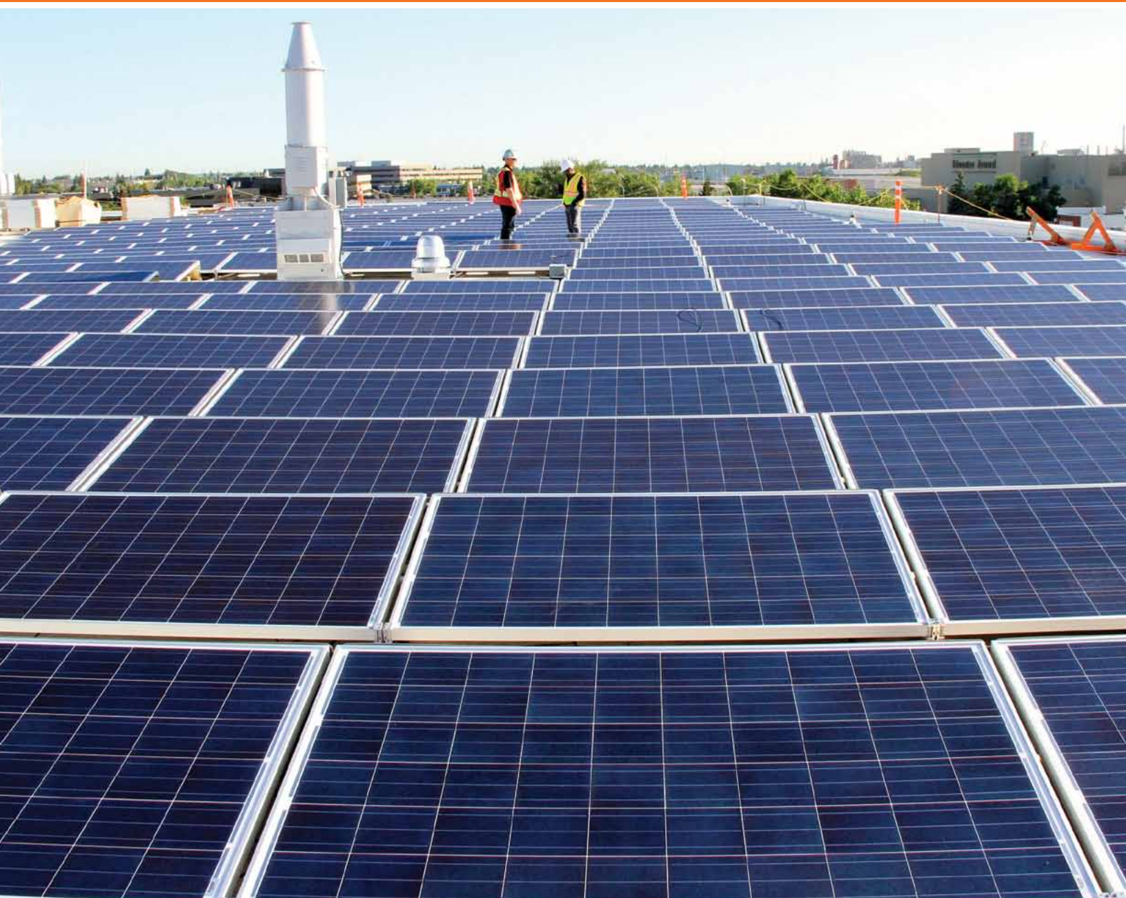
Photo: Solar array in Edmonton, Alberta.
