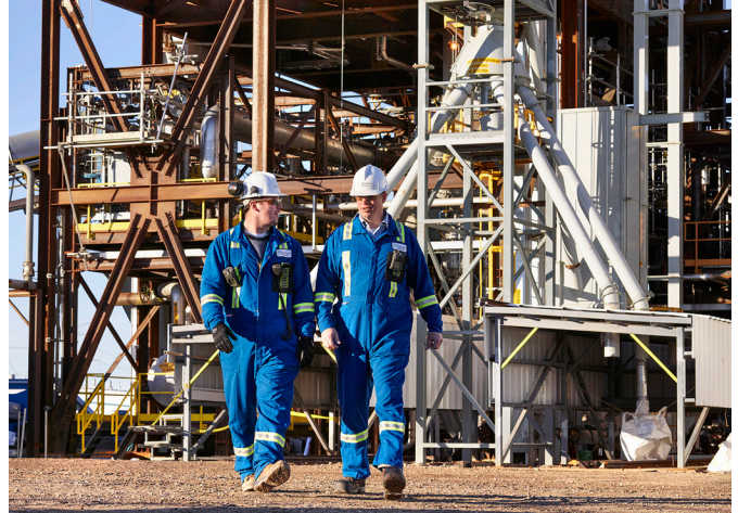
Energem's waste-to-fuel facility in Edmonton
